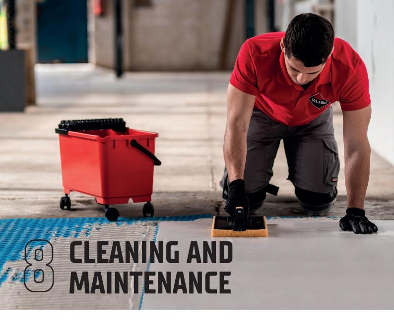
Once the tile installation and grouting operations have been completed, the surface of the ceramic material usually shows traces of cement in the form of a film or small accumulations. For the perfect elimination of these remains and dirt in general from the work, the use of specific slightly acid descaling detergents is recommended.
