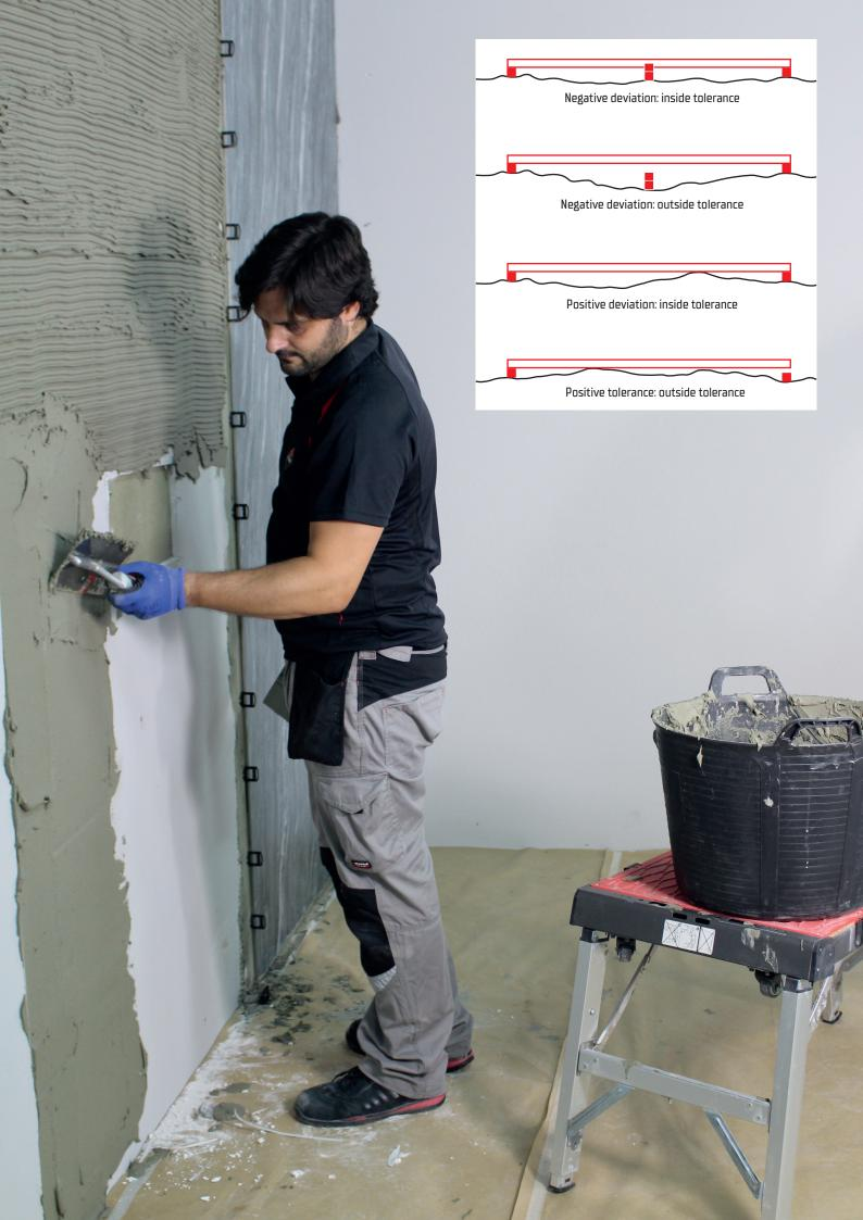
In order to achieve a good adhesion to the installation surface, it is necessary to prepare a solid firm surface, for which it will be necessary to proceed to a thorough cleaning or descaling of the surface to avoid adhesion problems or chemical reactions.
