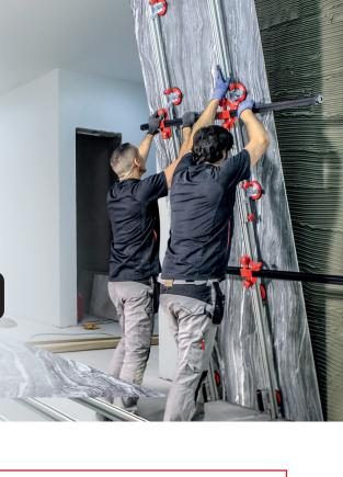
Large format ceramic tiles must be handled with extreme care, checking the space we have for maneuver and previously removing any object that may interfere with the movements of the piece.
