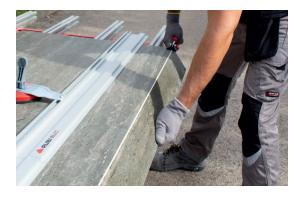
To finish the cut, the edges of the tile will be slightly sharp or irregular, we must finish them by beveling them with special discs or diamond pads to avoid accidents.
