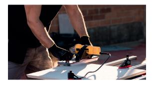
We must have the piece well seated on the table to carry out these works since they must be homogeneous along the entire edge of the large format ceramic tile.
