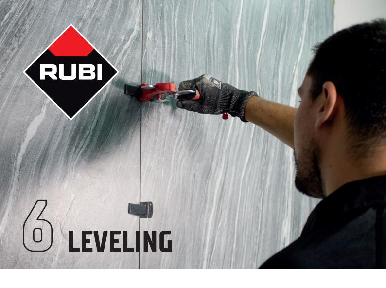
When we place a large format ceramic tile, with its thin thickness, it is possible that it is difficult to achieve an even finish with the adjoining pieces. This must be avoided at all costs in order to achieve the best finish, and we have an easy solution with the leveling systems.
