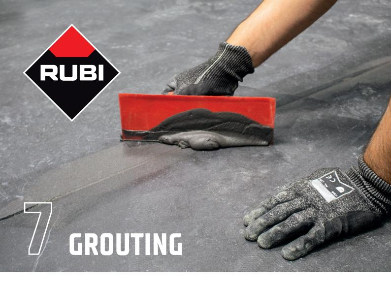
It should be noted that the base substrate is usually a continuous surface subject to contractions and expansions caused by thermal changes, structural movements, the effects of water or humidity, chemical reactions, or the shrinkage of the cement itself. For this reason, a perfect grouting guarantees that these natural movements of the substrate are not transferred to the tiled surface.
