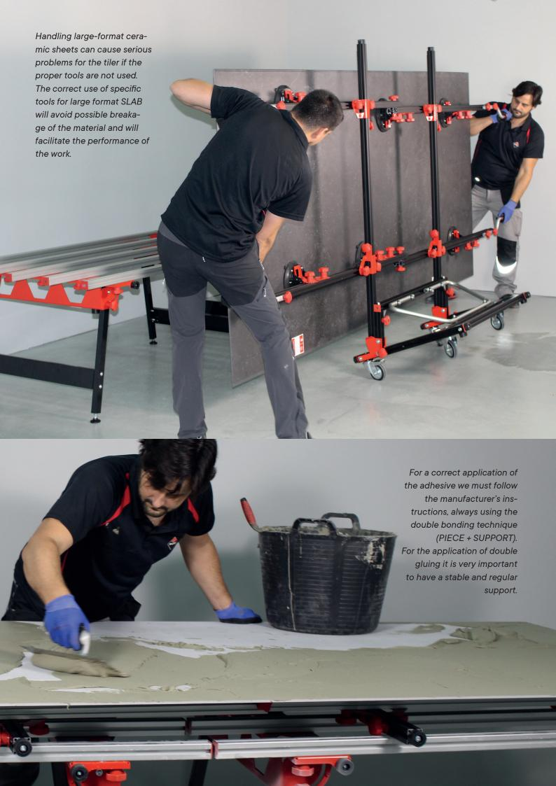
The adhesive should be spread in straight grooves, without fanning or curving, and parallel to the short side of the tile to reduce the distance the air will travel until it exits the ends of the tile.
