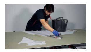
It is also correct to apply the "smearing" technique, which involves applying the adhesive with the smooth side of the notched trowel on the back of the tile, exerting light pressure on the ceramic.
