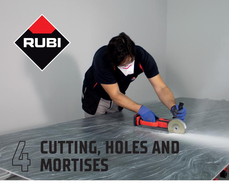
Although priority should always be given to the installation of complete pieces, it is inevitable that cuts will have to be made to adapt the piece to the installation space.
